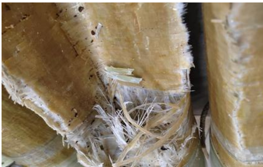
Fig. 1. – Photographs of fractures in hybrid glass-basalt-plastic pipes
